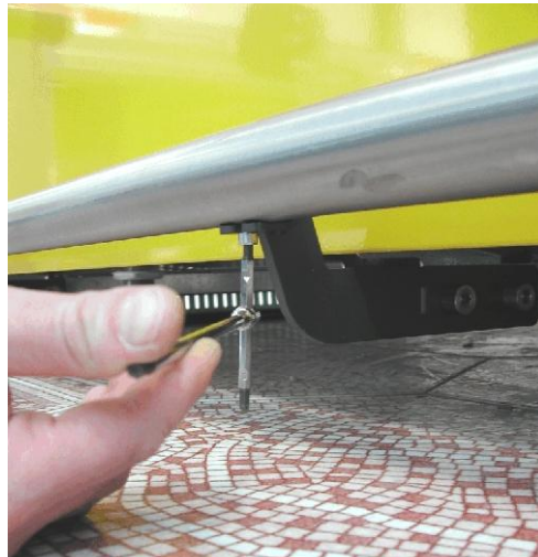
Fixing of the stainless steel tube onto the support brackets
